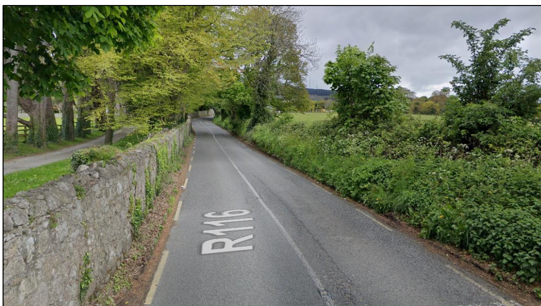
Figure 2-9 - Ballybetagh Road R116 Typical Road Section (source google maps)
